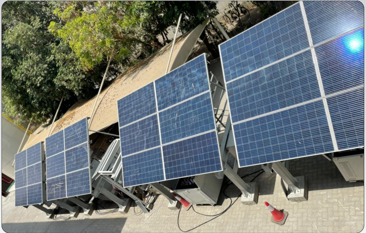
4KW Off-Grid Solar Power System for RTU(6 Days Autonomy), Emerson, Basra Oil Company, Iraq
