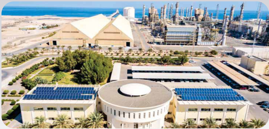
Omifco - 59 kwpc on-grid roof top solar power system Location: SUR Sultanate of Oman
