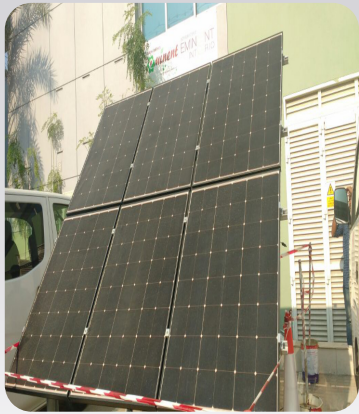
Yokogawa Solar Power System 2kWp- for RTU SNOC, Sharjah
