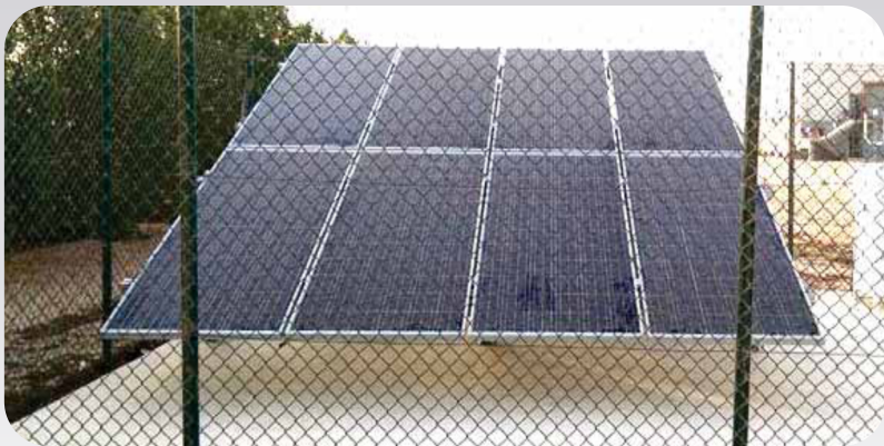
Enduser: Nawah Energy Company Location: Barakah nuclear power plant, Abu Dhabi. System: 2.4kwpc solar off - grid system
